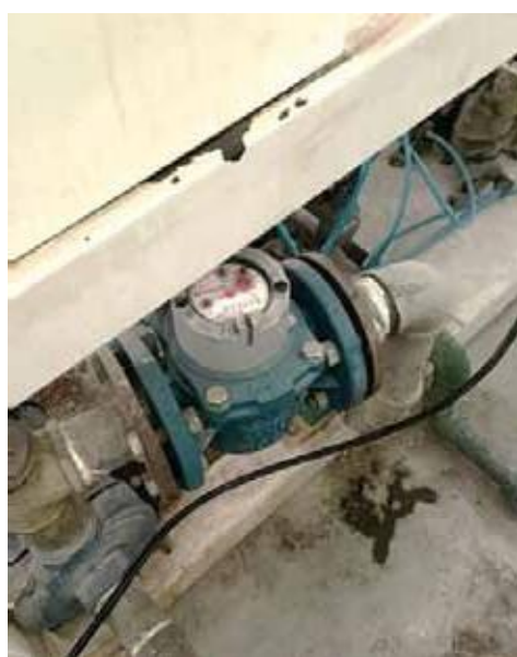
Meter to measure recycled water used at glue kitchen – BP MPak Sdn. Bhd.
